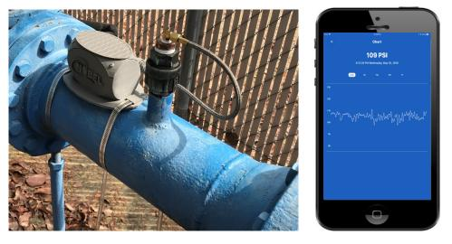
Figure 2-15. Example of Nobel Systems Water IoT – Pressure Monitoring
